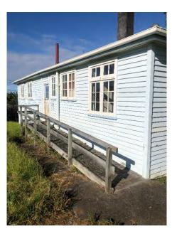
At the back door, the steps remain although a timber ramp has since been constructed over them. The ramp has been poorly built and never painted and is in poor condition. At the front door, there is some evidence of the steps settling with a gap opening between the steps and the rest of the building.
