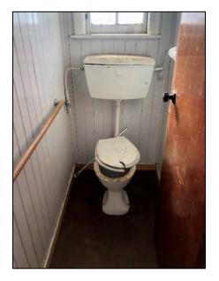
Area where plasterboard has been removed, exposing original tongue and groove linings (left) and toilet with tongue and groove boards still in place (right).
