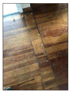
The floors comprise tongue and groove boards and generally appear to be in good condition. The timber is believed to be matai. A saw cut in the floor may have originated when the building was relocated, although the floor boards on either side of the cut do not match.
