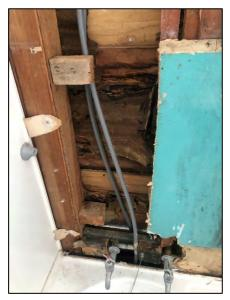
Areas of decayed weatherboards. The timber framing in these areas should be checked.
