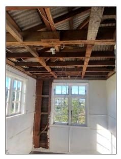
Areas of roof and ceiling framing. Note original timbers and later recycled material.
