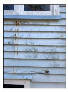
Cladding defects included decayed weatherboards (left), rusting grilles and decayed corner boxes (top right) and rusting soakers (bottom right).
