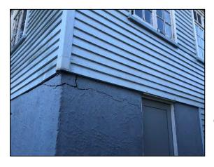
Crack in foundation wall at south corner.
