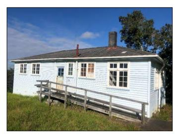
Rear side of building. Note corrugated asbestos cement roof and remnant of earlier lead flashing at the base of the chimney. Note also plastic spouting.
